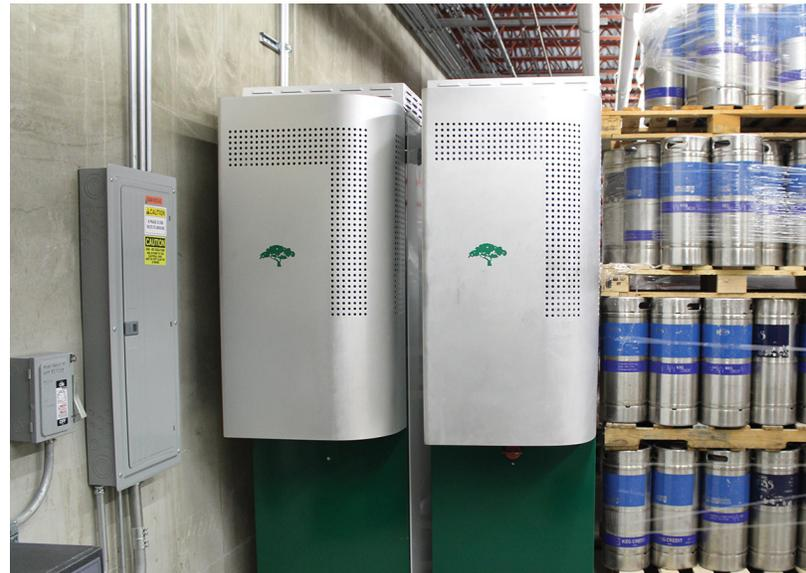
A 30 kW/60 kWh GridSynergy system, located in the basement of Mike Hess Brewing's North Park brewery, mitigates spikes in power demand caused by daily operations.
